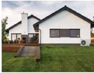
Air Source Heating
